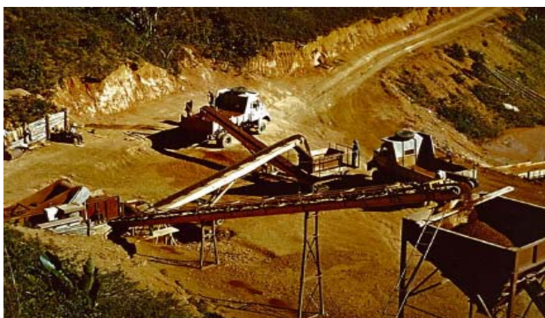
Figure 5.2. Washed bauxite production.
